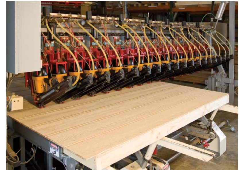
A BETTER WAY TO BUILD. Panelization wastes less; creates stronger, straighter, tighter walls; and goes together quickly at the site. Overall, it's better than stick building.
