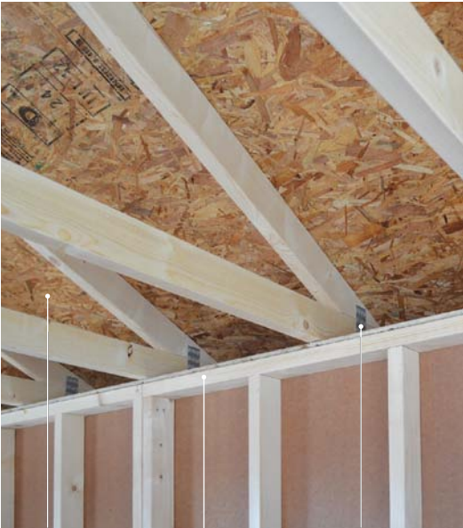
OSB roof sheathing 2"x4" bottom cord Metal truss plate
